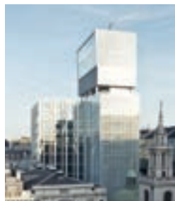
Cover: Rothschild's New Court Office. The site has been home to the Rothschild family business in London since 1809. © 2013 Hufton + Crow.
